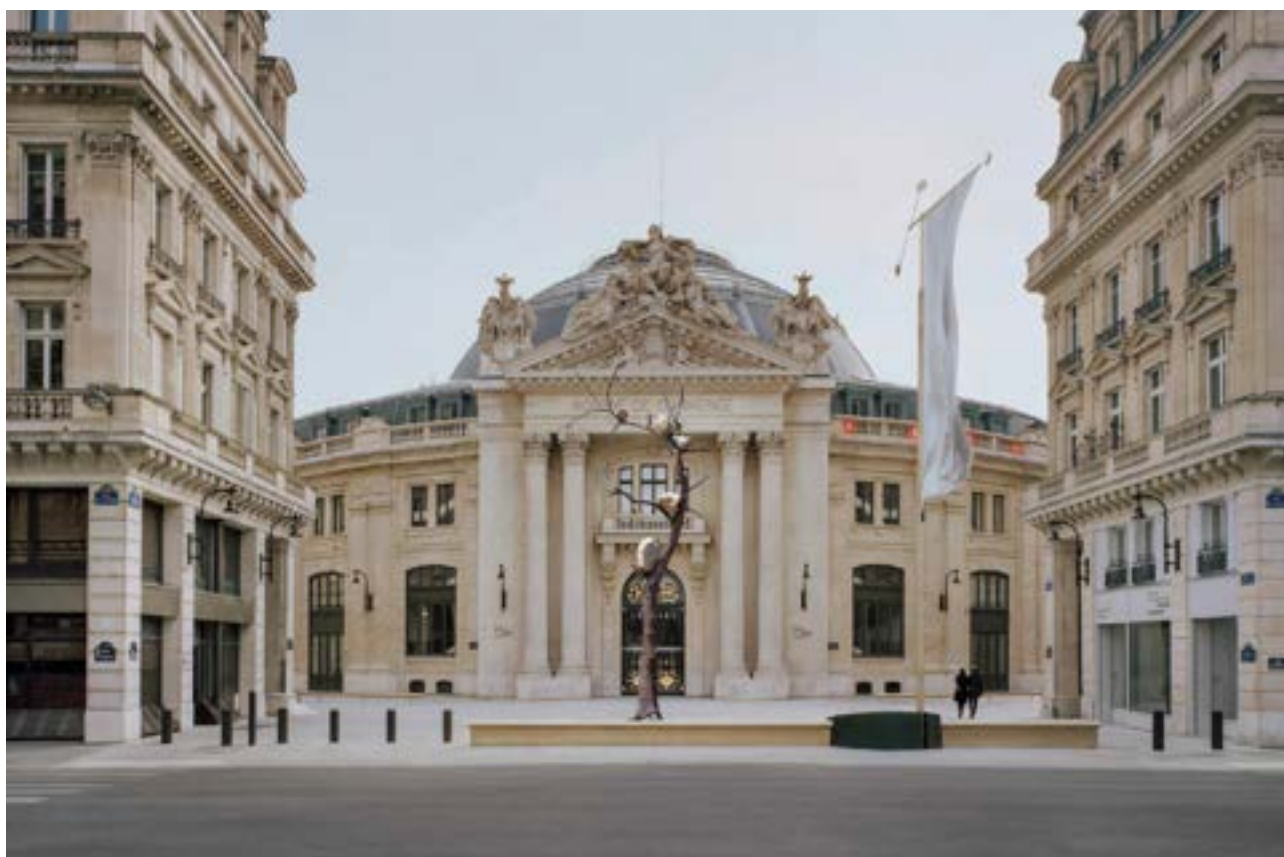
Simulation of an exterior view of the Bourse de Commerce – Pinault Collection with the works by Giuseppe Penone and Mario Merz. © Pinault Collection.
